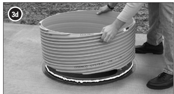
Carefully slide the riser onto the adapter.
