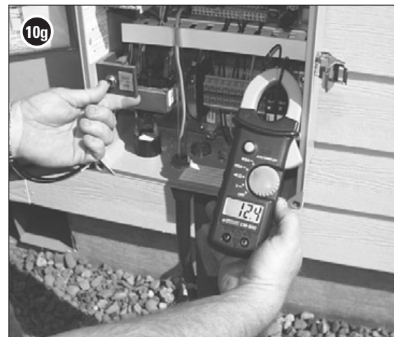
Measure amperage.
