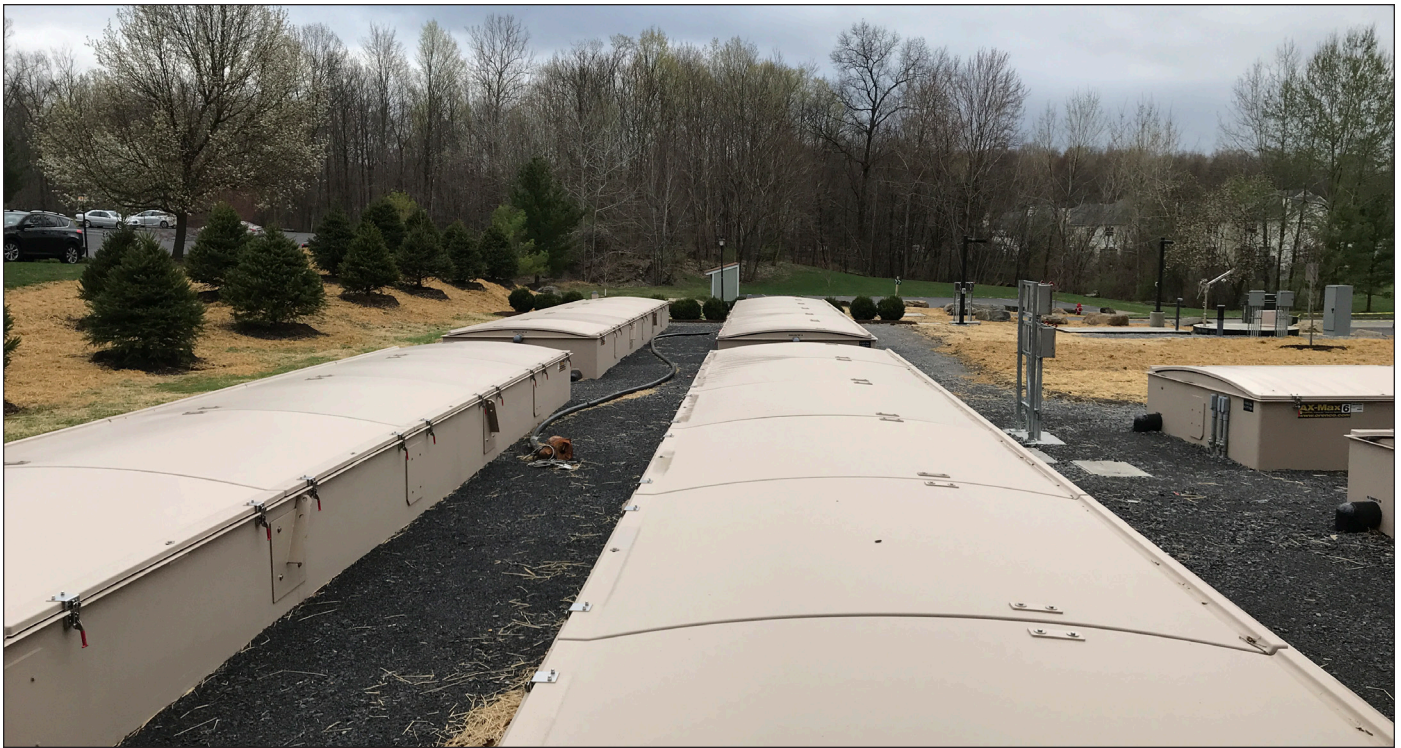
The AX-Max uses a passive, attached-growth treatment process that is inherently stable and has minimal operation and maintenance requirements. The Max also minimizes noise and odor, making it "neighborhood-friendly." (Photo courtesy of the Dutchess County Water and Wastewater Authority.)
