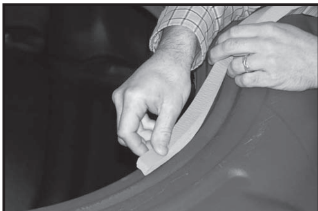
FIG.2 Apply Gasket
